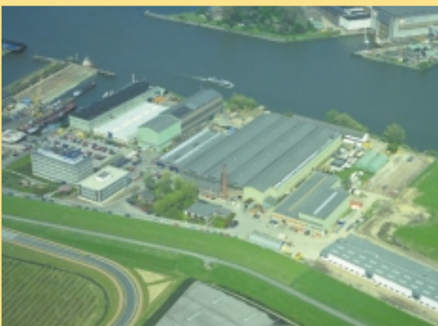
HMA Power Systems factory
