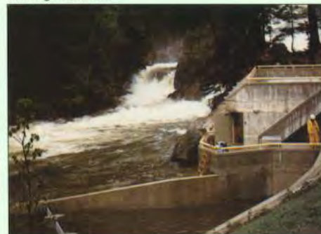
Fig. 13 The Weeks Falls Hydro Site, Washington, U.S.A. Another Kvaerner Hydro Power engineered site with Brush generation.
