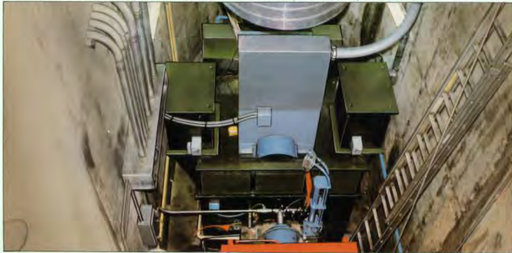
Fig. 10. Valley Falls Hydro-electric installation New York, U.S.A. incorporating a 2.967 MW, 900 rev/min (overspeed 2900 rev/min), 4160 V, 3 ph, 60 Hz. Brush generator supplied through Kvaerner Hydro Power Inc.
