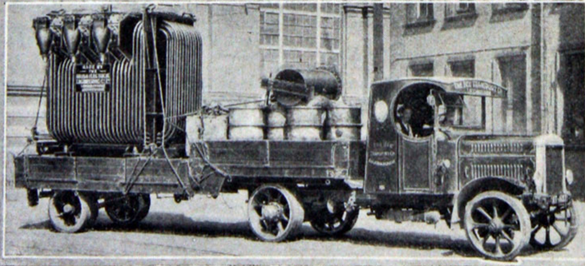
HEAVY HAULAGE BY ROAD. Twenty tons is the total weight of this load—a transformer with the necessary insulating oil in barrels—on a Carrimore six-wheeler. It is seen leaving the works of the Brush Electrical Engineering Co., Ltd., Loughborough.
