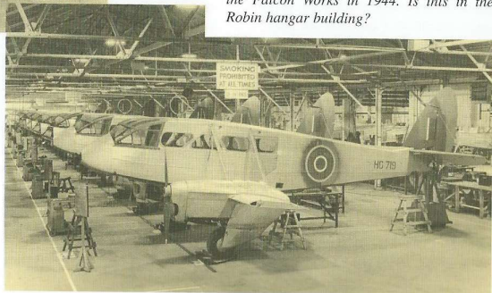
The De Havilland Dominie assembly line at the Falcon Works in 1944. Is this in the Robin hangar building?
