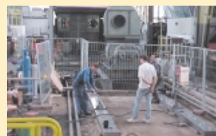
Work in progress on HMA's new test bed
