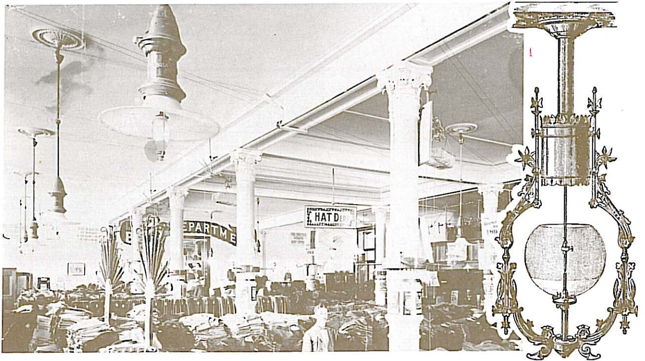
A Brush arc lamp and arc lamps in the Brill Brothers Store in New York City.
