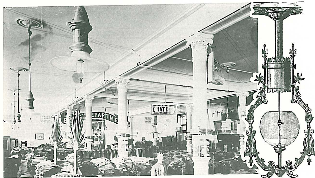
A Brush arc lamp and arc lamps in the Brill Brothers Store in New York City.
